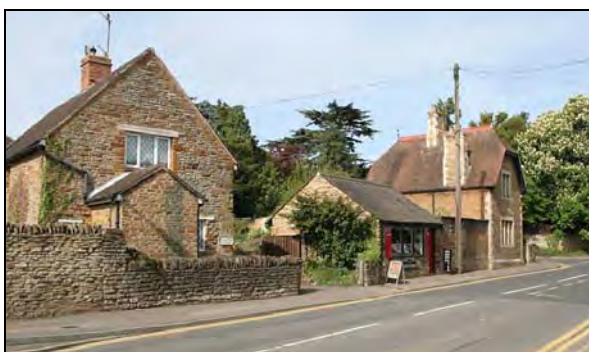
Nos 47-51 Main Road
