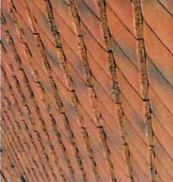
TYPE R2 Artificial clay appearance roof tiles by Marley Eternit - Ashmore Interlocking Double Plain Tile -colour Olde English Dark Red or similar approved.
