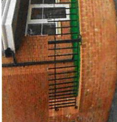
TYPE B2 1.2m high boundary wall - metal fence on top of a brickwork plinth - in black. Brickwork - IBSTOCK Wylam Olde Blend or similar approved.
