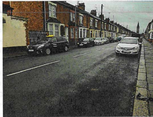
Southampton Road 2.30pm on a weekday in June
