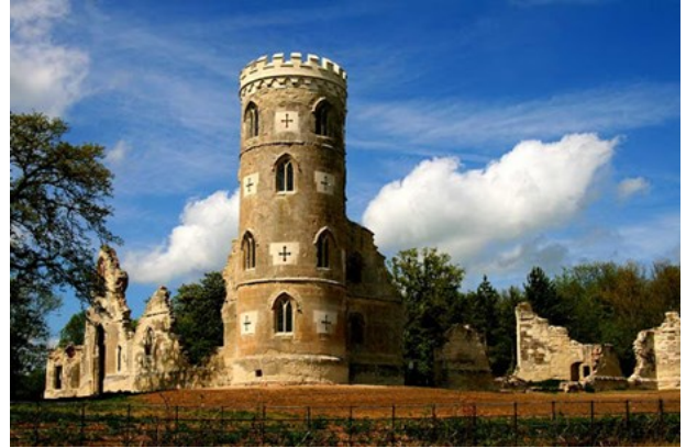
Wimpole's Folly – Peter Dann, Consulting Engineers, Cambridge
